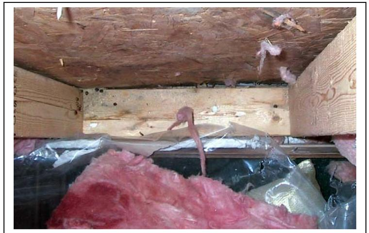
Do the math: The temperature indoors is 75° F. The temperature outdoors is 95° F. The outdoor humidity is 70 percent RH. The temperature behind the drywall is 76° F. By using a psychrometric chart, you find the incoming air dew point is 84 °F. This is what the six-mil plastic interstitial vapor barrier looks like after you remove the drywall. The inside of the surface of the plastic is where the condensation will occur.
